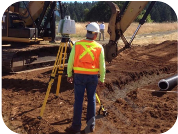
Addressing Challenges in Automation in Highway Construction, Part II
