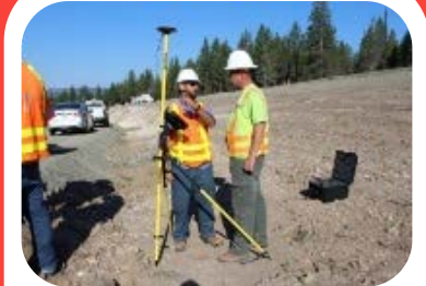
Construction Inspection for Digital Project Delivery
