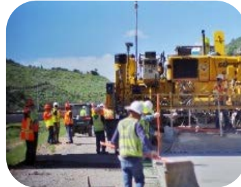
Utilizing 3D Digital Data in Highway Construction
